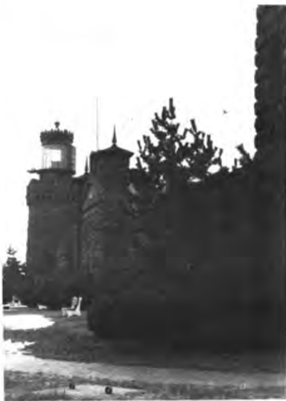
Exterior of Twin Lights (NJ) showing the south light tower and, at lower left, one of the four original concrete guy anchors for the old wooden mast.
